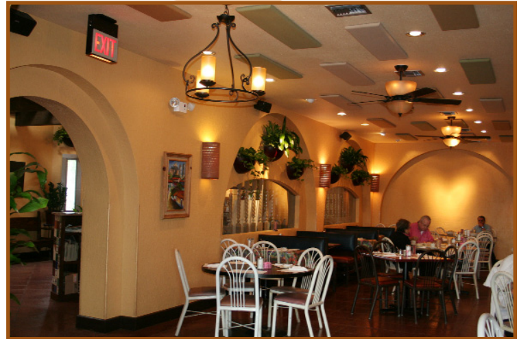
The panels on the ceiling of the restaurant pictured at the top of this article are 12" wide x 48" long x 1" thick Fabric Wrapped Fiberglass panels with radius (rounded) edges and Guilford Anchorage fabric facing (Colors: 2130 Vanilla, - 2034 Straw, & 2048 Green Olive). They are mounted to the ceiling with the two part clip system – and there are four clips on each panel. The colors were chosen by the customer to fit the existing color scheme of the room.
